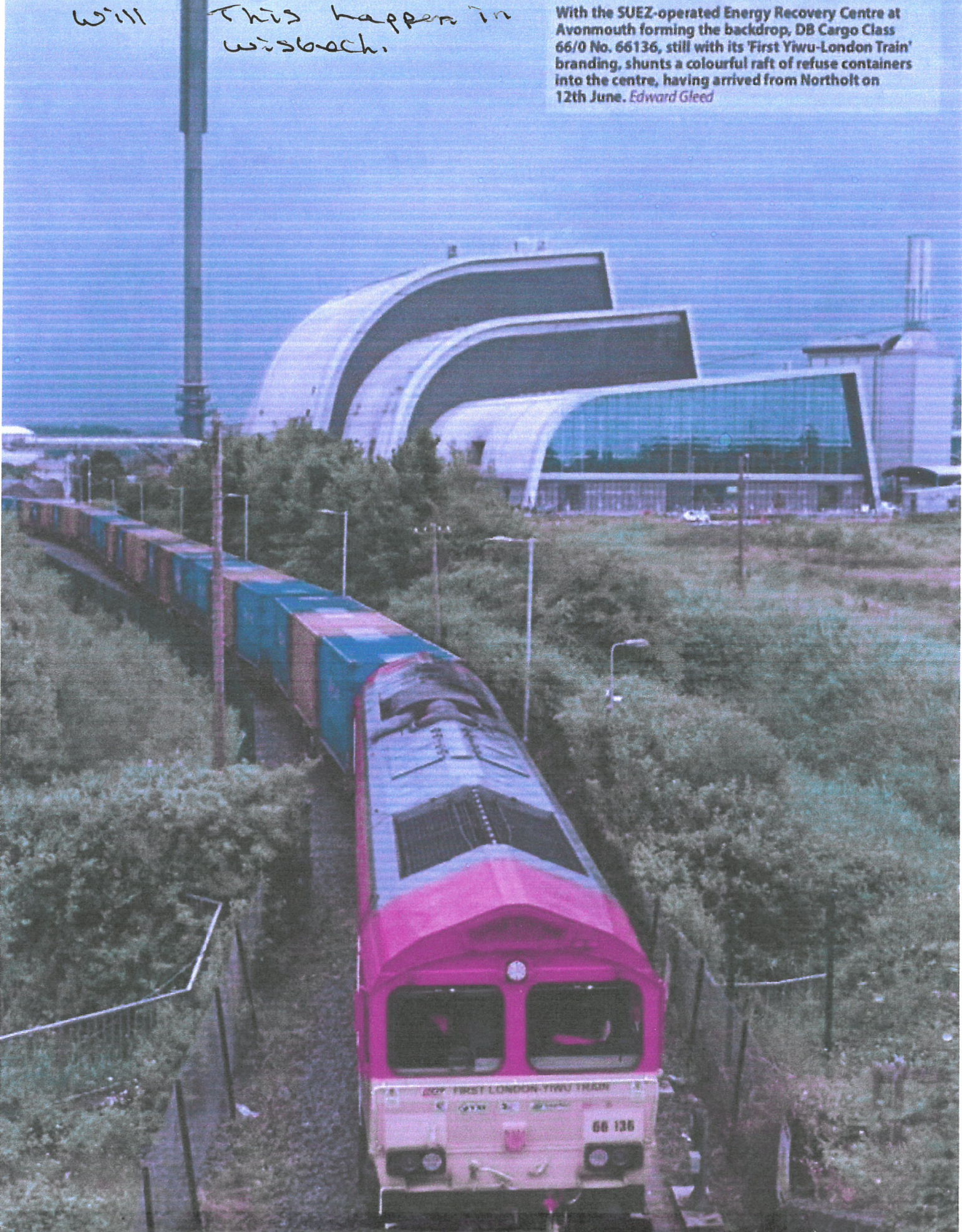
This is the Incinerator (sorry, Energy Recovery Centre - sounds so much better!) in Avonmouth on the outskirts of Bristol. It is 125 miles from London and receives regular trainloads of London waste for incineration. Wisbech is only 100 miles from London, so with a reopened railway could easily become the dumping ground for London's rubbish!
